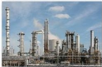
化工厂 Chemical Plant
